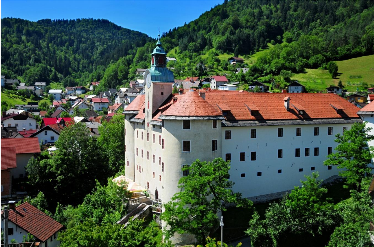
PHOTO 1: GEWERKENEGG CASTLE - BUILT AS THE ADMINISTRATIVE BUILDING OF THE IDRİJA MERCURY MINE (AUTHOR: DUNJA WEDAM)
